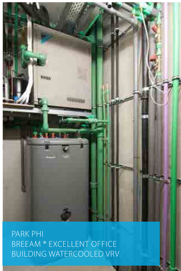
EIFPAGE OFFICE, VRV IV WITH CONTINUOUS HEATING
